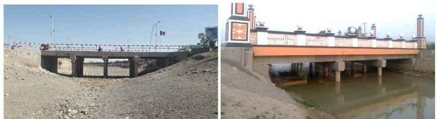
Figure 2. Existing bridges on Zahirshahi canal.
