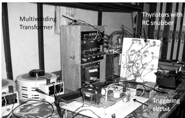
Figure 12. Complete set up of the multilevel grid tie inverter.
