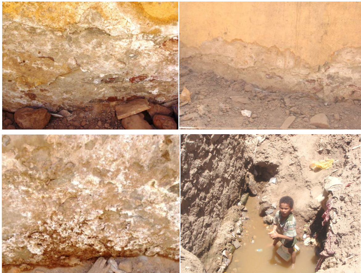
Figure 12. Salt crystals cause the building materials to split, flake and crack (Khor Awada and El Sail areas).
