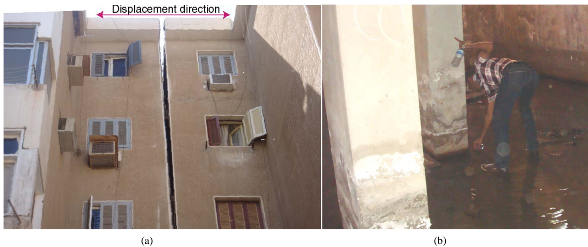
Figure 14. Groundwater rising and their environmental impact: (a) Displacement occurs between two buildings, (b) Example of flooding buried basements of many buildings. (a) El Aqad; (b) Aswan stadium.
