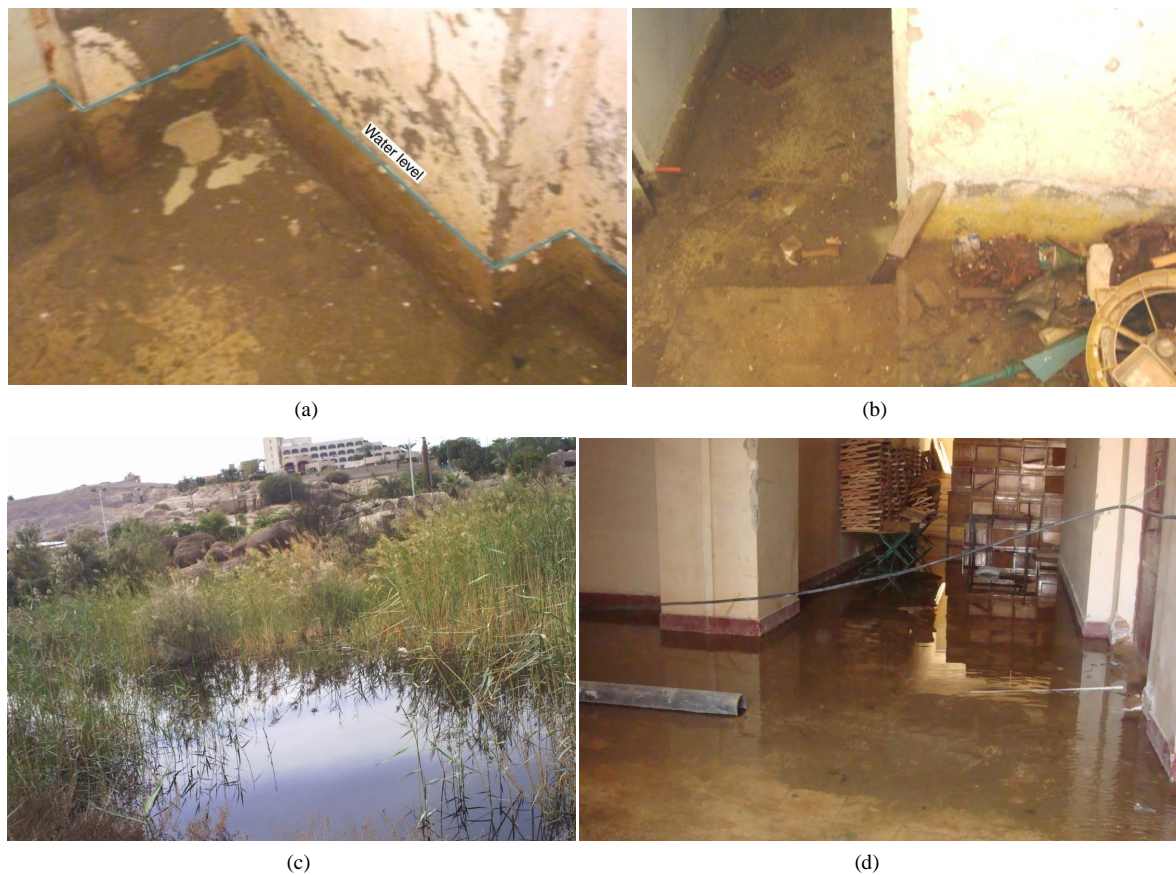
Figure 2. Rising groundwater level affecting areas: (a) KhorAwada, (b) El-Seil, (c) Phatic graves area, and (d) Aswan stadium.
