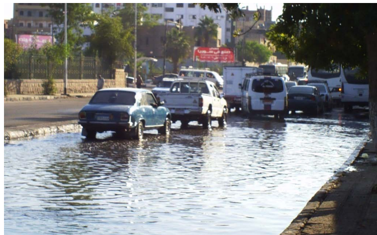
Figure 10. Rash of sewage network system on streets.
