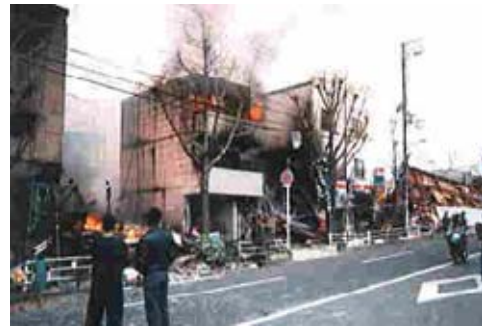
Figure 1. Fire after gas leakage.
