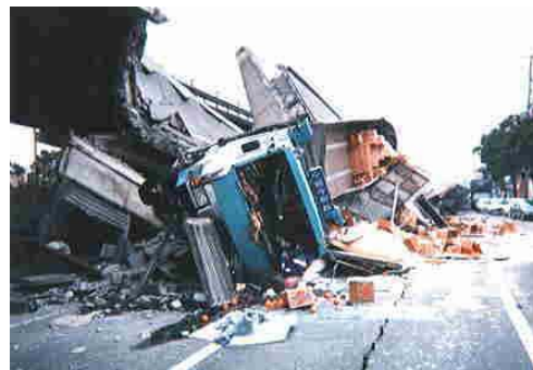
Figure 2. Road damage after earthquake.
