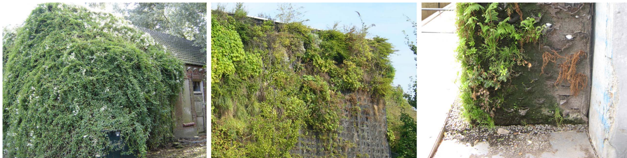
Figure 3. Examples of possible damages due to the lack of maintenance and to design mistakes.
