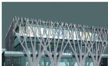
**Figure 7.** Bearing skeleton of walls of Jiangwan Cheng, Chongqing, China [13].
