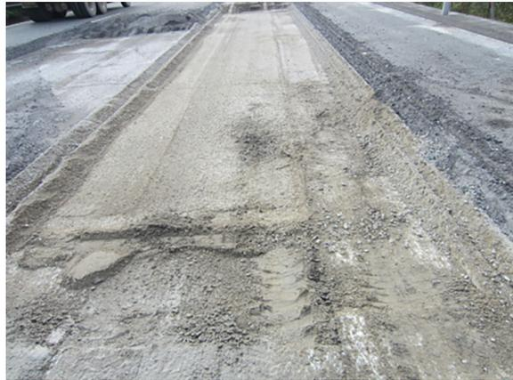
Figure 24. Photo of top subbase at K2900 + 605 - K2900 + 610.
