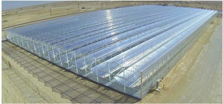
Figure 5. Photo of the enclosed trough system facility installed in the Amal oil field, Oman [17].
