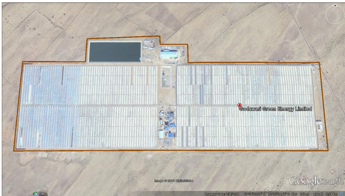
Figure 5. Google earth image of 50 MW solar thermal power plant, Nokh, Rajasthan [30].
