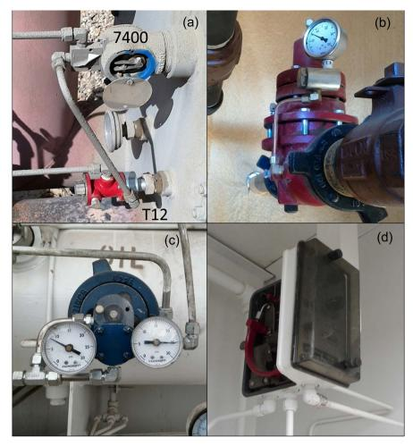
**Figure 1.** Example PCs encountered in this study: (a) WellMark 7400 IPC level and Kimray T12 temperature IPC; (b) Kimray back pressure regulator IPC; (C) WellMark 6900 level controller IPC; and (d) Fisher<sup>™</sup> 4660 high-low pressure pilot CPC with side cover removed.
