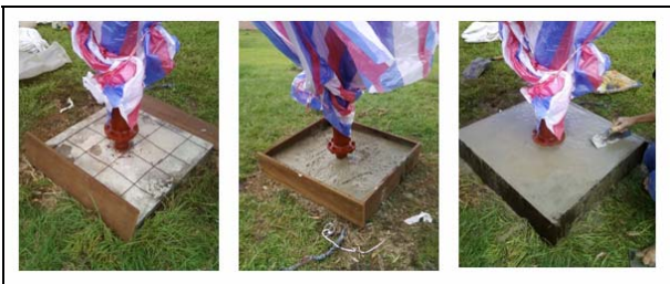
Applying an extra layer of concrete to the base
