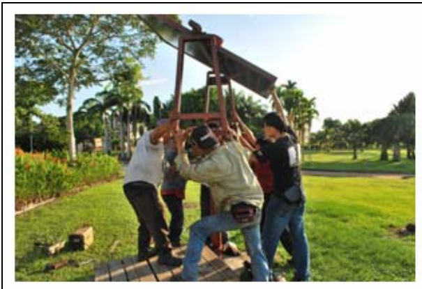
The frame being attached to the column
