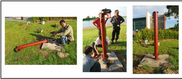
Base of the column is welded and the column being set up
