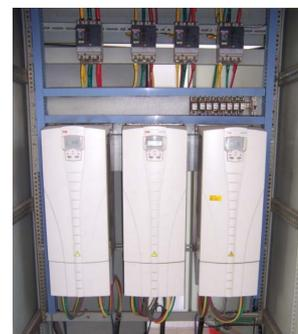
Figure 4. Frequency conversion power counter.
