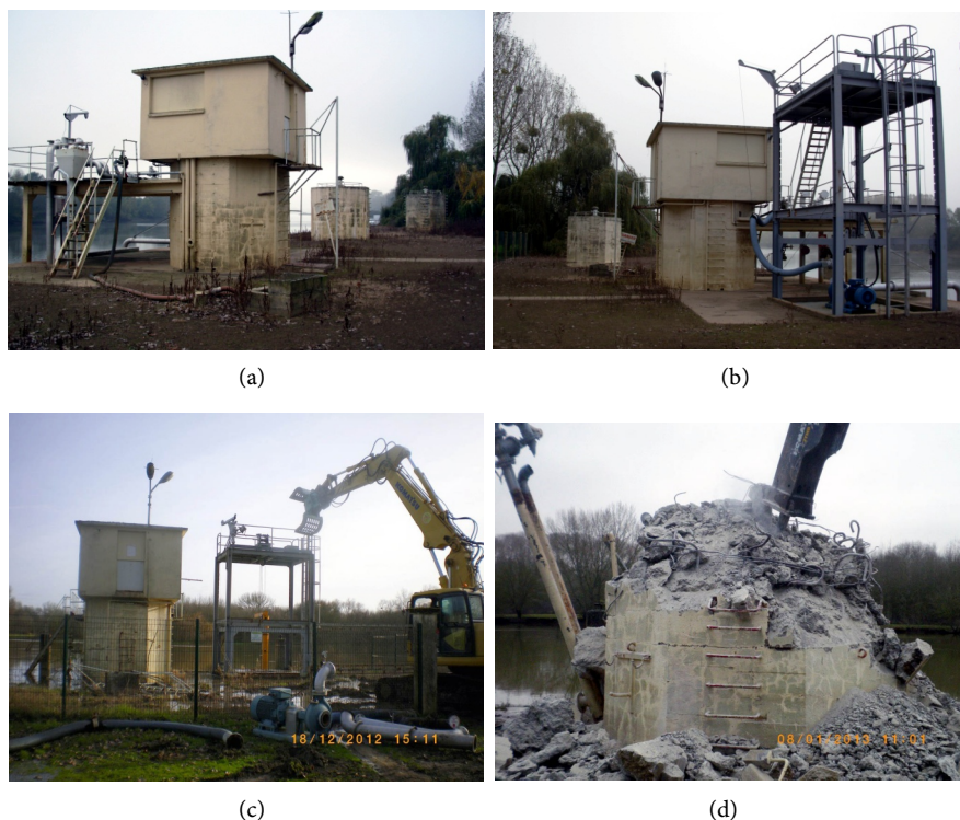
Figure 9. Pumping station and bollard c demolition—(a) side view, on the left the added metallic platform with oil discharging tubes, on the foreground right the columnar bollards d, e (courtesy Mr F. Guillaume, 07 th November 2006); (b) side view, on the foreground left the columnar bollard b, on the right the metallic platform with oil discharging tubes (courtesy Mr F. Guillaume, 07 th November 2006); (c) platform and pumping station demolition (courtesy Mr F. Guillaume); (d) bollard c demolition (courtesy Mr F. Guillaume).
