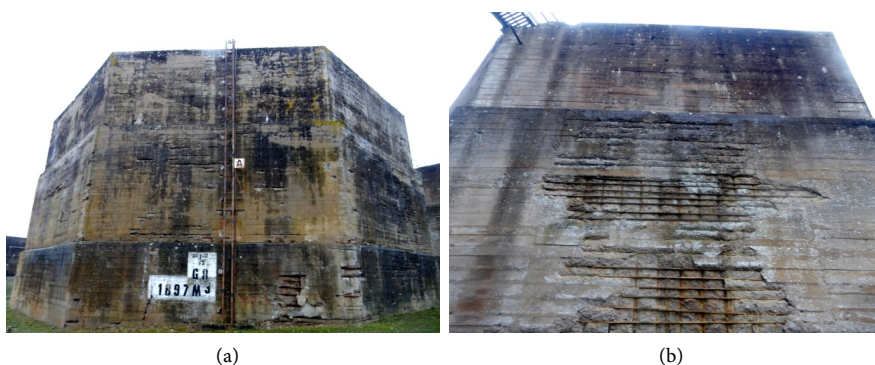
Figure 13. Octagonal wall A—(a) three steps external structure with white board; (b) local concrete superficial failures.
