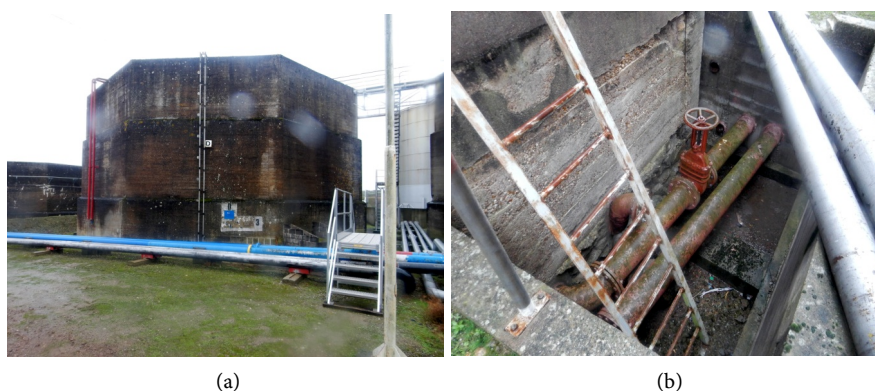
Figure 14. octagonal wall D—(a) external structure with white board covered by a square, blue board; (b) concrete pit with connection pipes.
