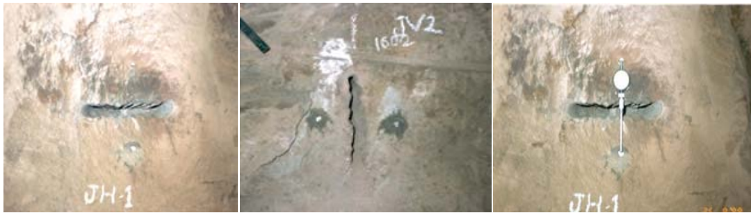
Figure 2. Slots made by jack hammer drilling and convergence measurement by deform-meter.
