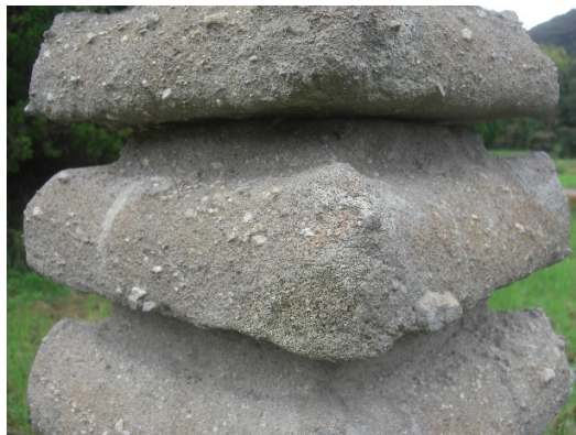
Figure 16. Restored and fixed part of the stone tower.
