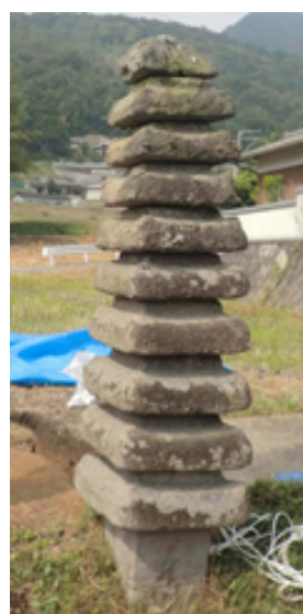
Figure 15. Stone tower made by tuff breccia before applying Aquo-Siloxane method.
