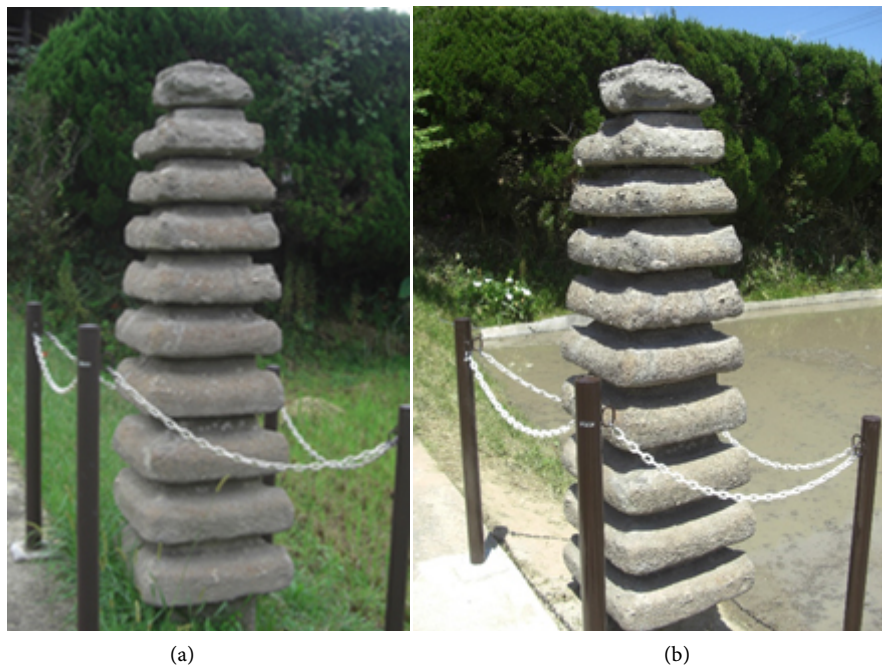
Figure 17. Stone tower after preservation treatments including Aquo-Siloxane treatment. (a) After one year; (b) After four years.
