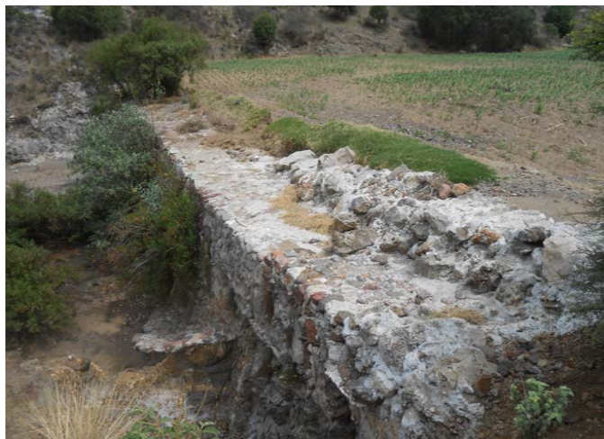
Figure 6. El Pedregal dam, spillway water curtain maintenance (Galindo 2015).
