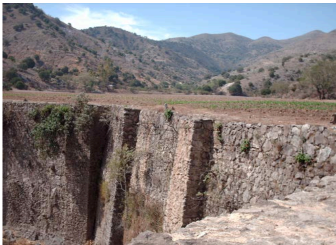
Figure 5. El Saucillo dam, spillway water curtain (Galindo 2015).
