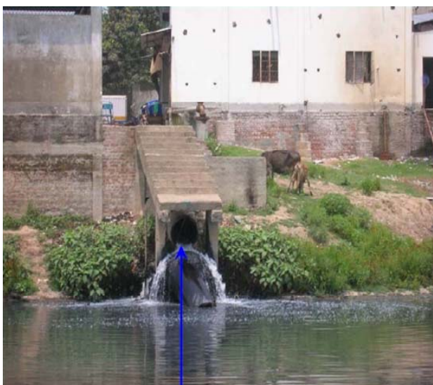
Figure 4. Industrial wastewater discharge in Turag river.
