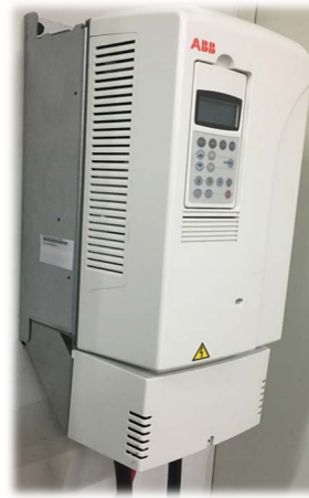
Figure 30. VFD—Variable Frequency Drive.
