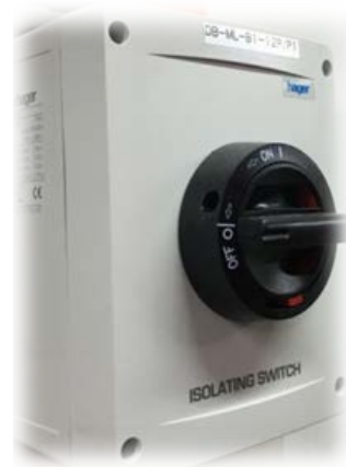
Figure 27. Utility AC input (3-phase power supply from laboratory distribution panel).
