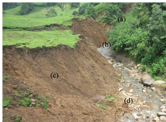
Figure 3. River bank erosion, in Gilgel Gibe catchment, causing sediments loading (d), and bank collapses (c) and performance of a vegetated bank portion (a) in diverting water flow (d), adapted from [21].
