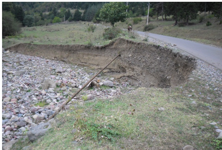
Figure 13. Sakire-Dviri damaged road.
