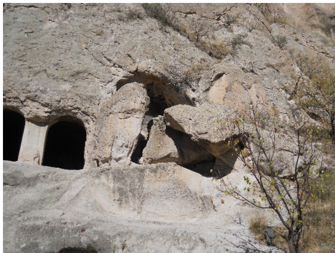
Figure 21. Rockfall processes in Vardzia complex.
