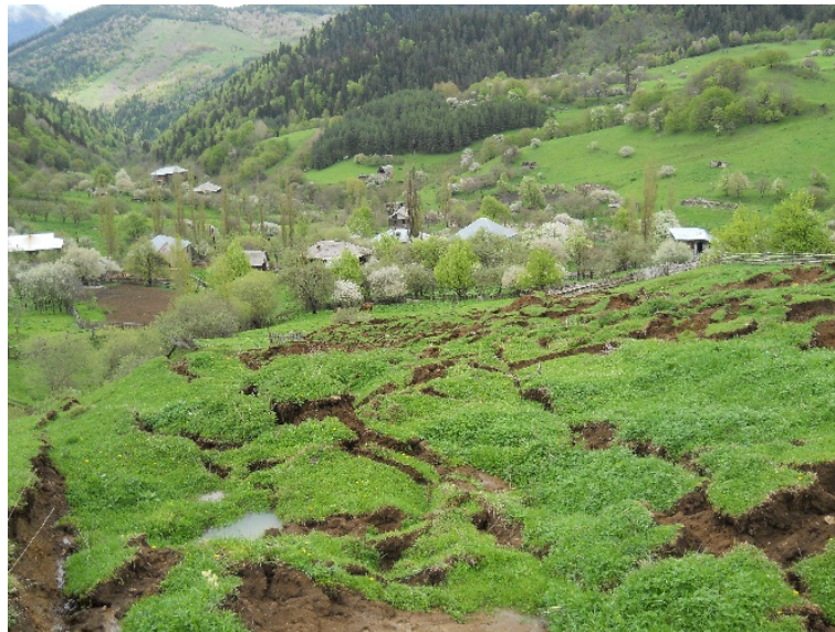
Figure 11. Village Didi Mitarbi landslide.
