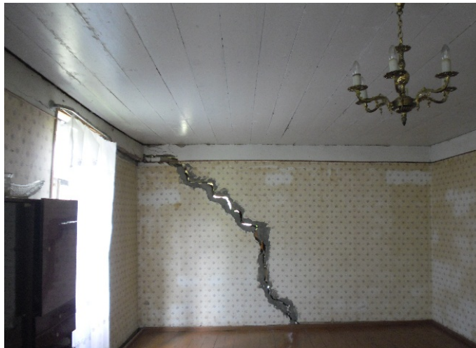
Figure 9. Village Dgvari, house damaged by landslide.
