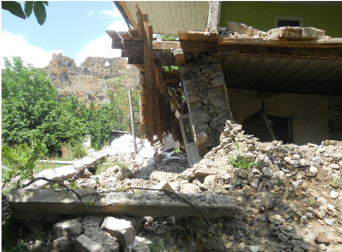
Figure 16. Village Gaghma-Atskuri landslide, destroyed house.
