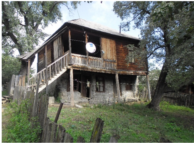
Figure 8. Village Dgvari, house damaged by landslide.
