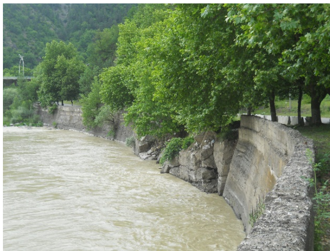
Figure 7. Riv. Mtkvari right bank erosion.
