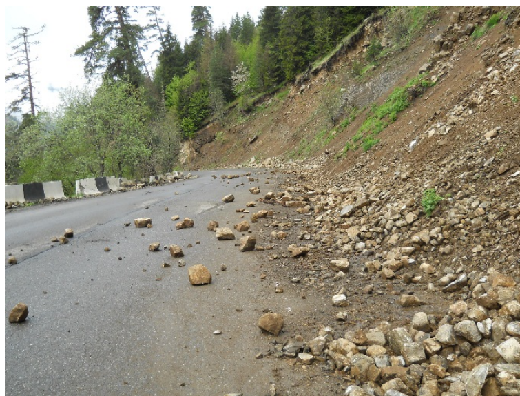
Figure 14. Rockfall (Borjomi-Bakuriani road).
