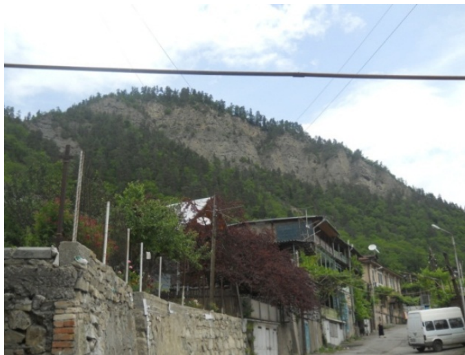
Figure 6. City Borjomi, rockfall area.
