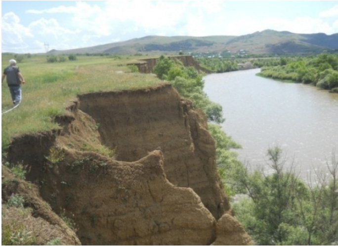
Figure 17. Riverbank erosion (Tkemlana-Sakuneti section).
