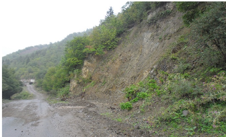
Figure 18. Rockfall (Chobiskhevi road).
