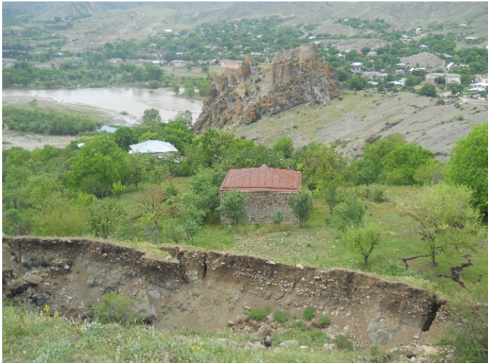
Figure 15. Village Gaghma-Atskuri landslide.
