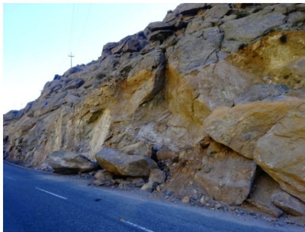
Facet no. 1 showing wedge failure.
