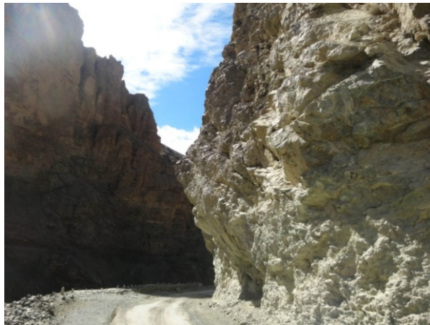
Facet 37 highly block and undercutting prone to toppling failure.
