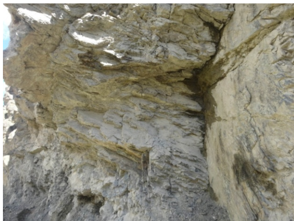
Highly fractured facet no. 58 showing damp area prone to failure.
