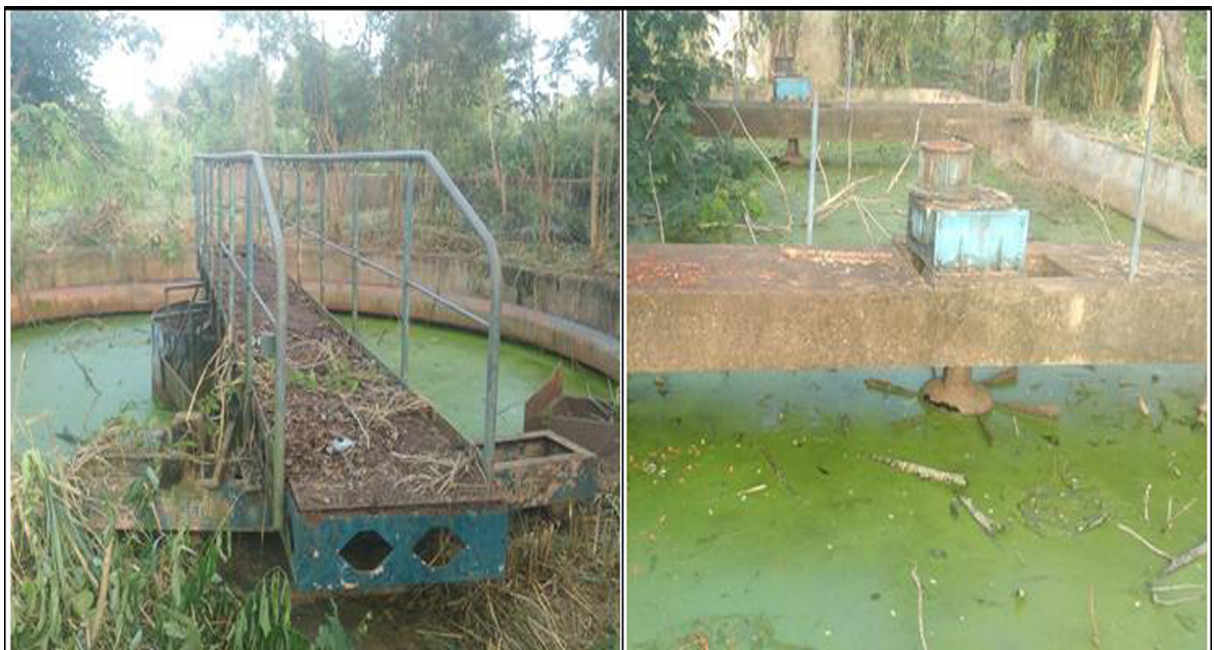
Figure 4. Inoperative wastewater treatment plant.
