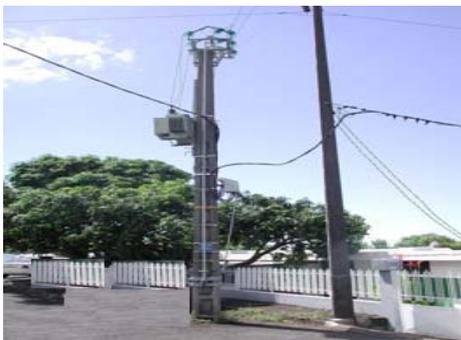
**Figure 1. Pole-mounted transformer substation.**
