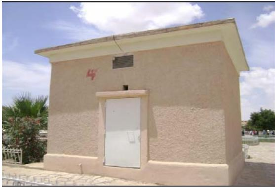
Figure 3. Masonry Substation.
