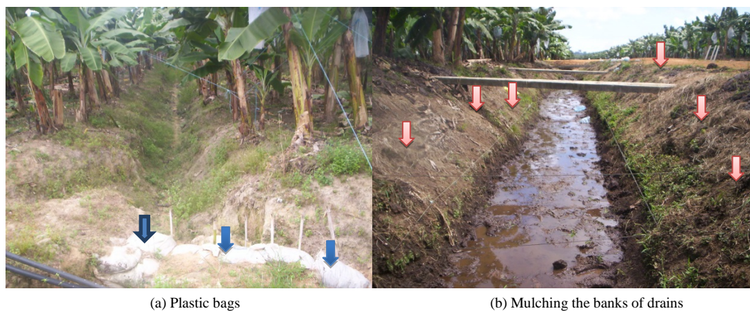
Figure 3. Some methods used in planting against erosion drains.
