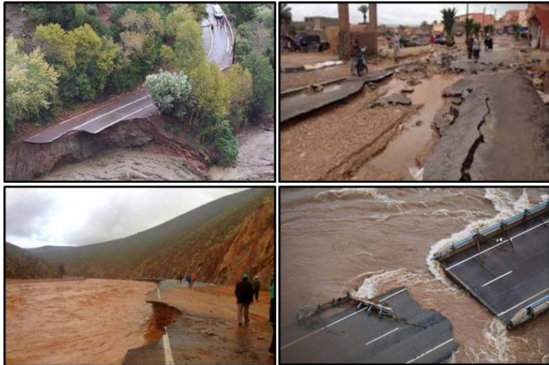
Figure 3. Destruction of road and bridge infrastructure in the Guelmim city region on 24 November 2014 (Photos from the web).
